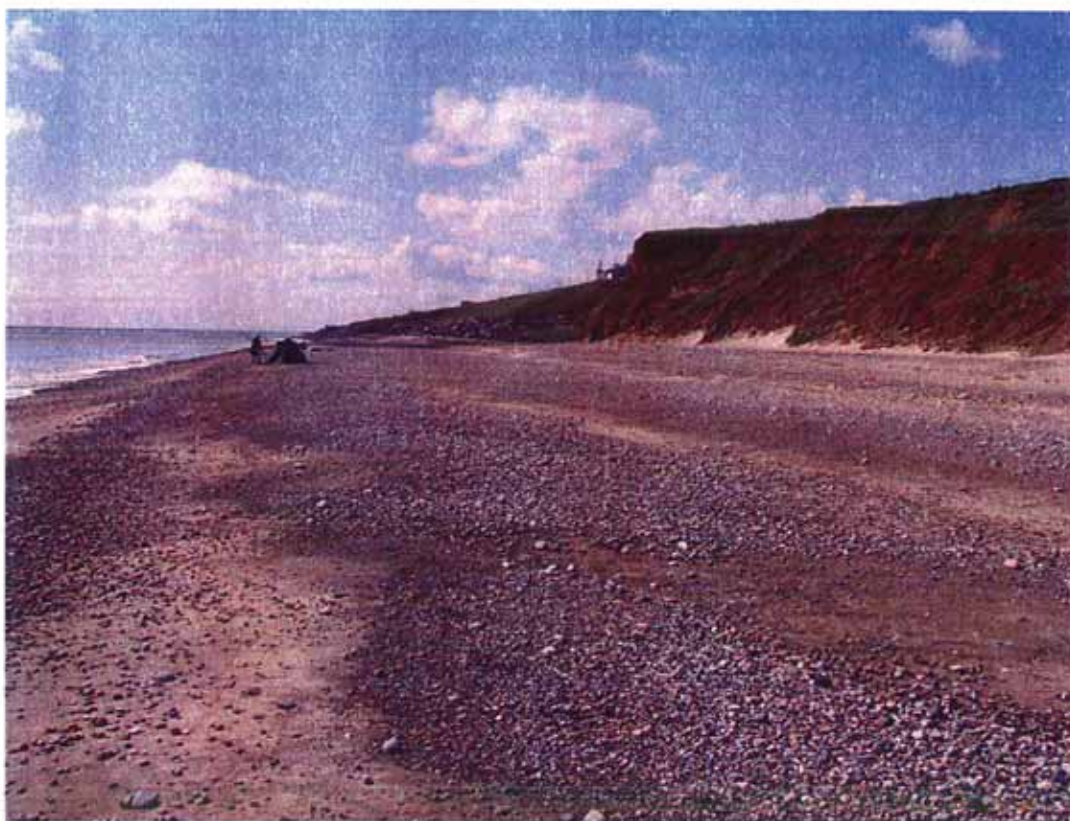
Plate 4 The natural cliff face north of the revetment looking south
