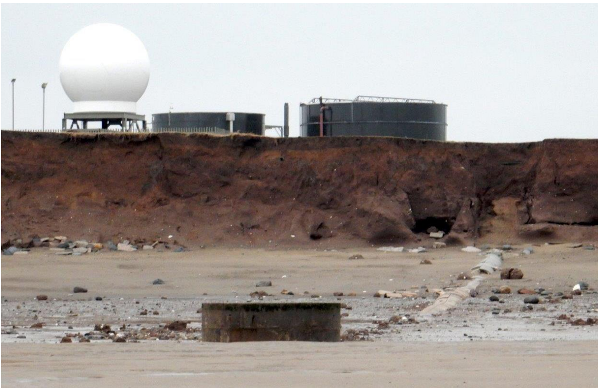
Figure 2017: 04 Construction shaft on the beach with exposed tunnel section and WwTW
